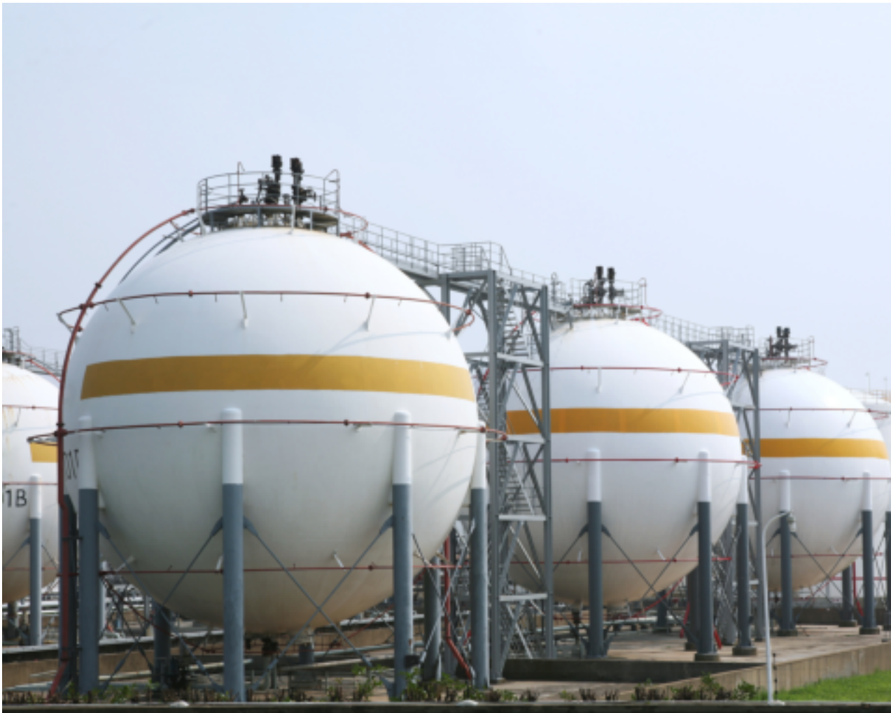
Natural gas tank
