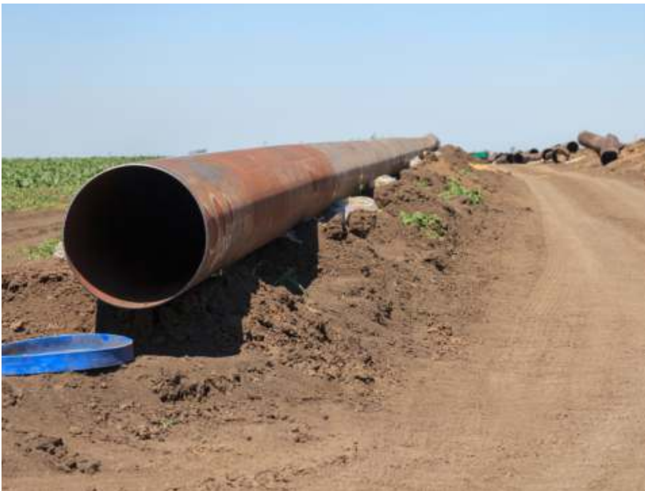
Gas pipeline construction, illustrative image
